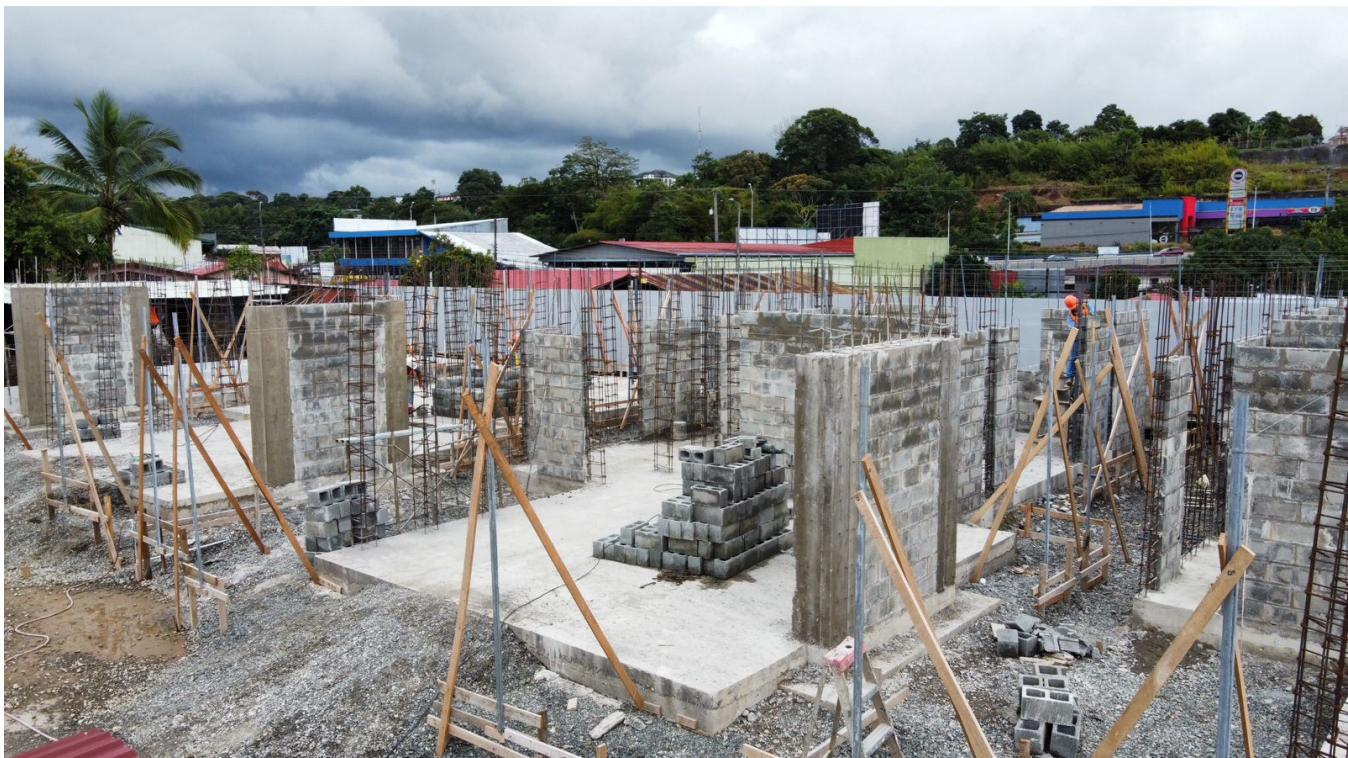
3. **\*Wall Reinforcement\***: During construction, metal or other reinforcements are inserted as needed to increase structural strength. This step is crucial to ensure the walls can support additional loads and withstand potential ground movements.
